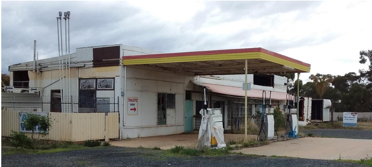
Abandoned petrol station: Norseman, WA. Image: B Gatton
